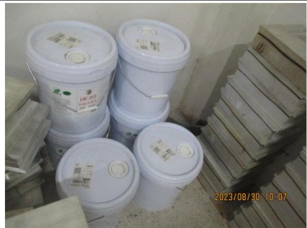
NC: Lack of MSDS and secondary containment.
